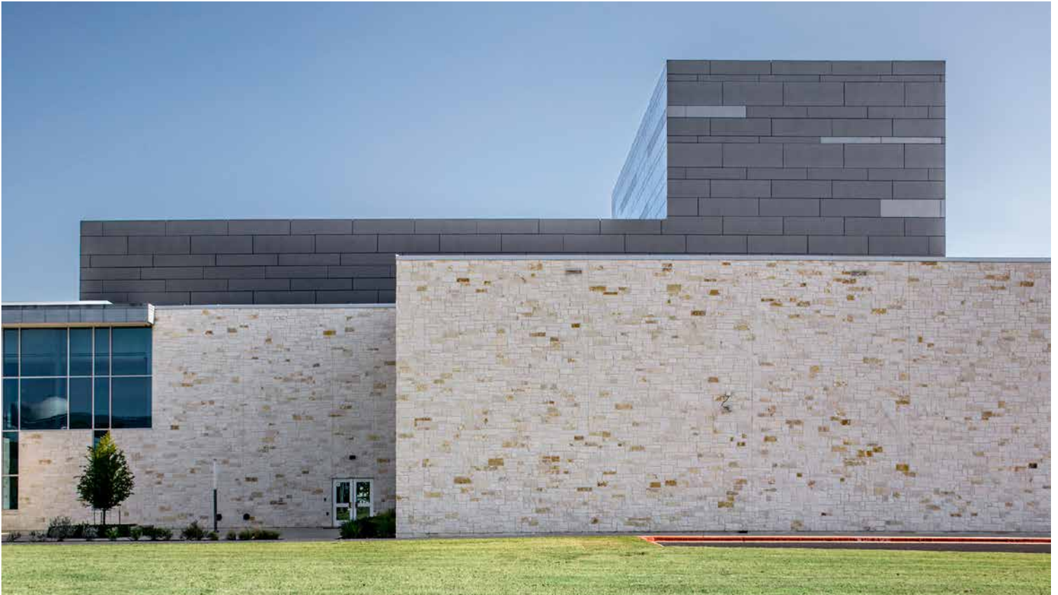
The building volume, comprising cubic volumes, is clad mainly with light natural stone and dark gray fiber-cement panels.
